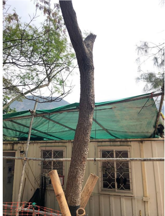
Photo 17: Trunk condition of G62/RT-07
