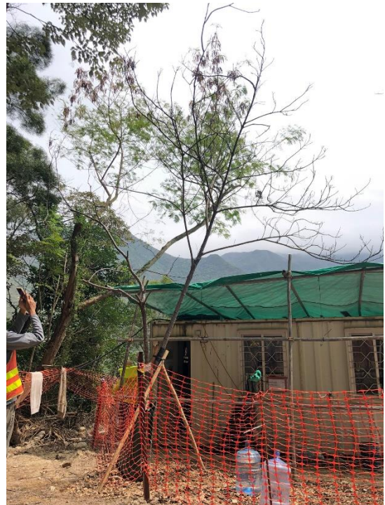
Photo 23: Whole view of G62/RT-08
