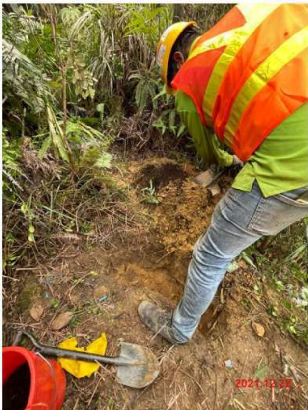
Backfilled with soil mix-A
