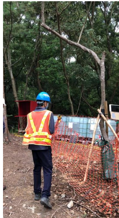
Photo 35: Trunk condition for G62/RT-07
