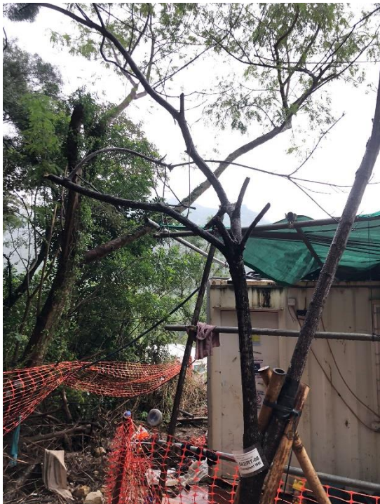
Photo 30: Crown condition of G62/RT-08
