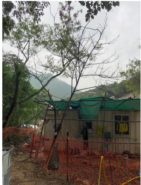
Photo 31: Whole view of G62/RT-08
