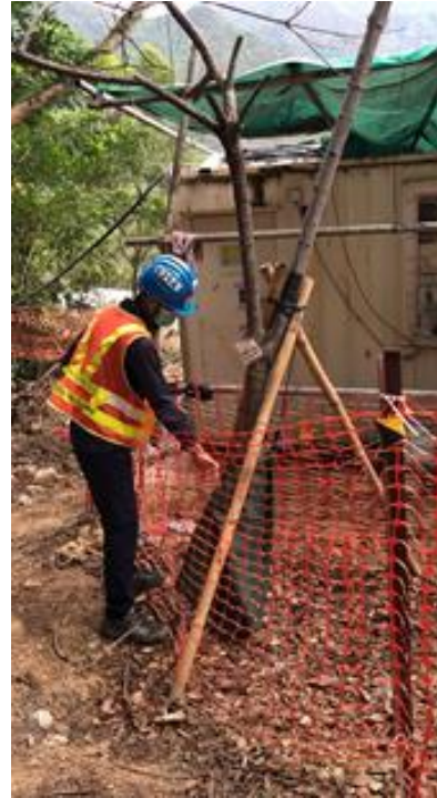
Photo 37: Trunk condition of G62/RT-08
